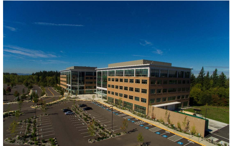
Fisher Creek 2 is one of the most energy-efficient commercial buildings in the surrounding Clark County, WA area, with self-dimming sustainable lighting and customized windows to reduce the energy used for heating/cooling.
